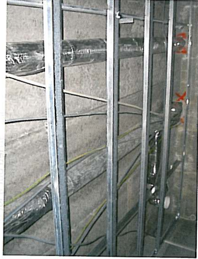
Ventilation ducting in suspended ceiling.
