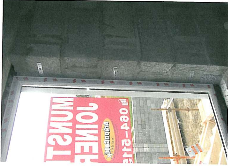
Window thermal bridging detail, including Polypearl infill.
