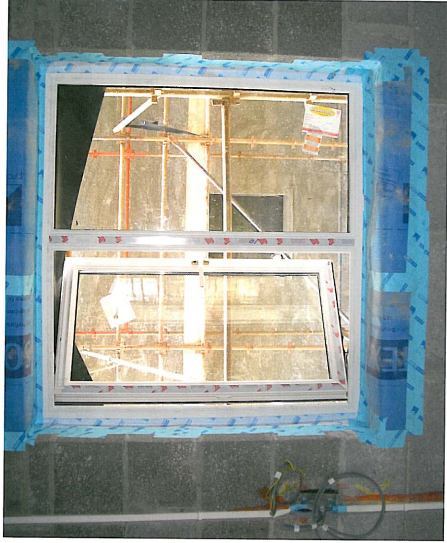
Airtight sealing of window on the Castlemagner site.
